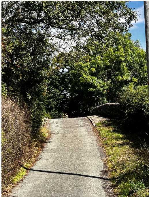
Approach to the bridge on The Grand Union Canal
