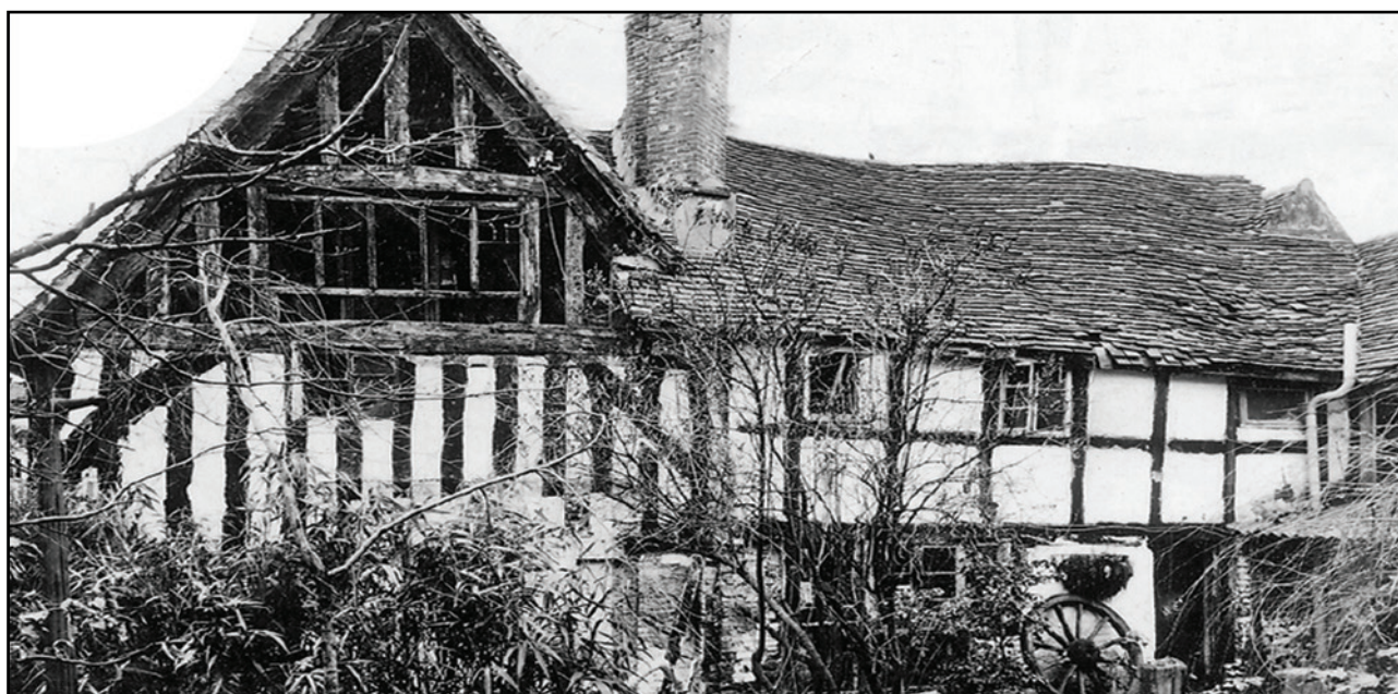
Chester House - before restoration and opening as Knowle Library, 1975
