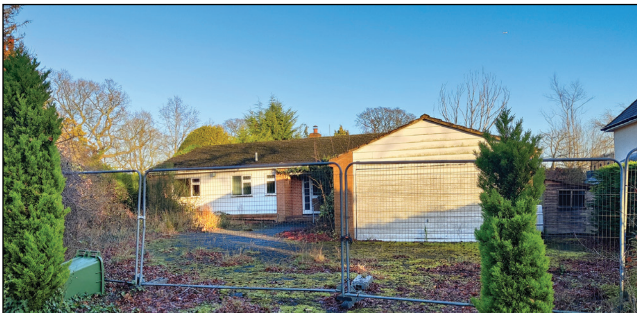
Proposed entrance to the Bloor Homes site by demolition of 51 Knowle Wood Road
