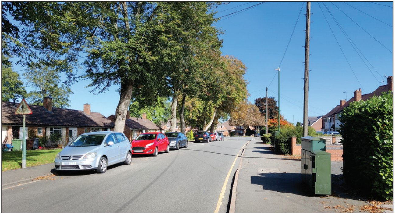
Straight run along Lodge Road, a temptation for speeding
