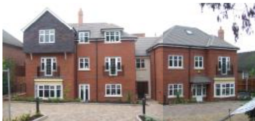
242 and 240 Station Road with BT Telephone Exchange on far right (Photo montage: David Bower)
