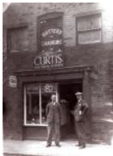
Curtis Electrical - Arthur & Vic
