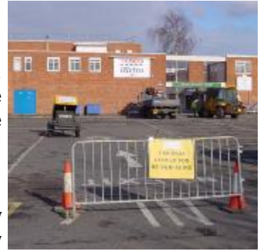
Shoppers' car park closed for work
