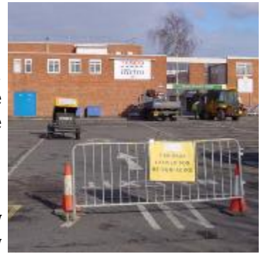
Shoppers' car park closed for work
